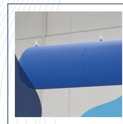
The **DHI TEXTILE** product line helps reduced maintenance times due to its lightweight durability. The material allows for easy washing, are non-flammable and available in a number of different colours to match your brand.
